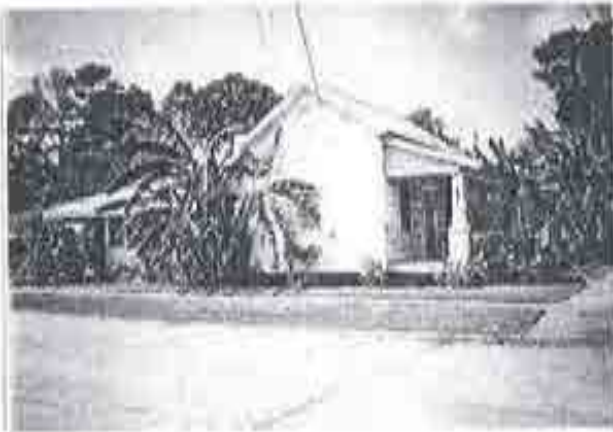
Between the Northbound and Southbound Thruway Near Mudd
