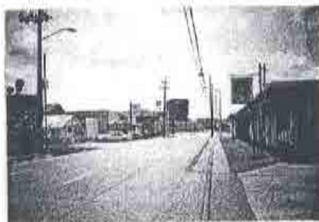
Looking West on 3 rd Street Toward the CBD Between the Thruway and Railroad
