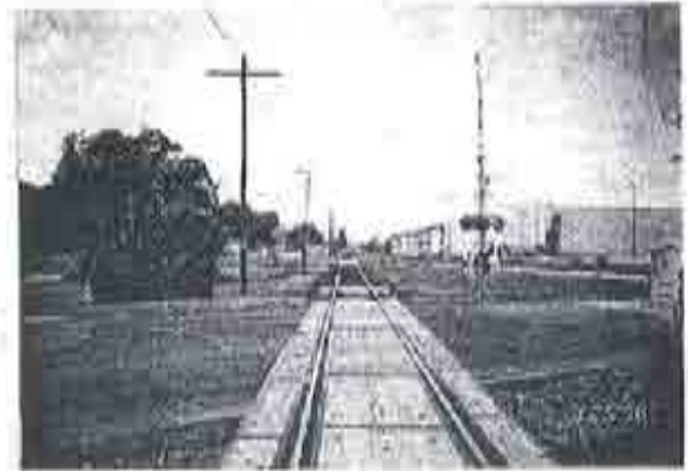
Adjacent to Union Pacific Railroad Looking North Near Taft
