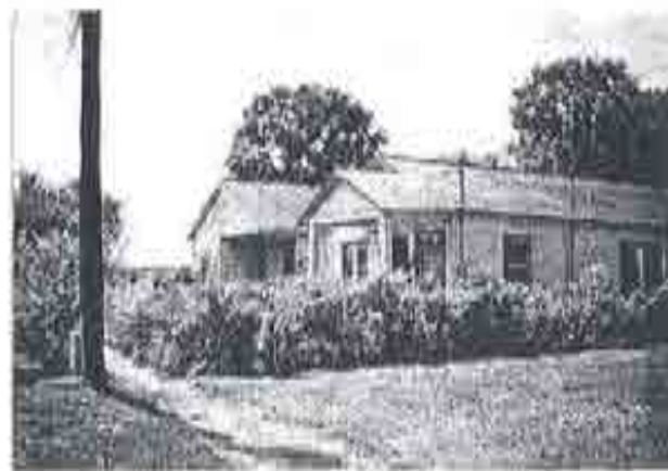
Between the Northbound and Southbound Thruway at 11 th Street.
