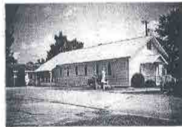
Christ The King Church on the Median Side of the Southbound Thruway Near Mudd
