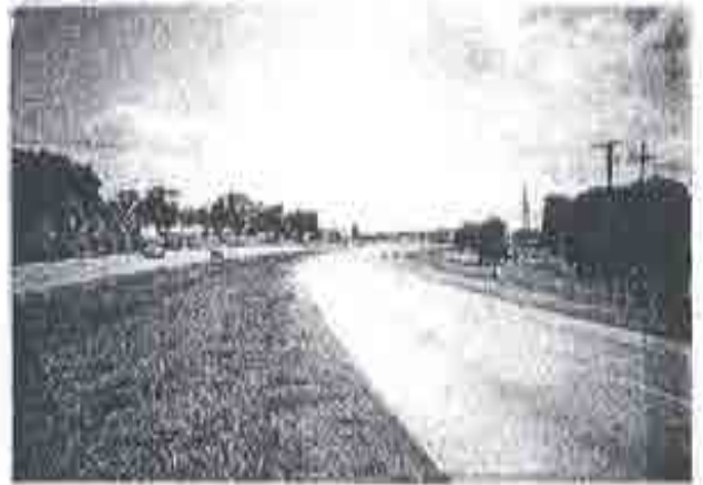
Looking South on the Thruway Flanked Both Sides by Beaver Park
